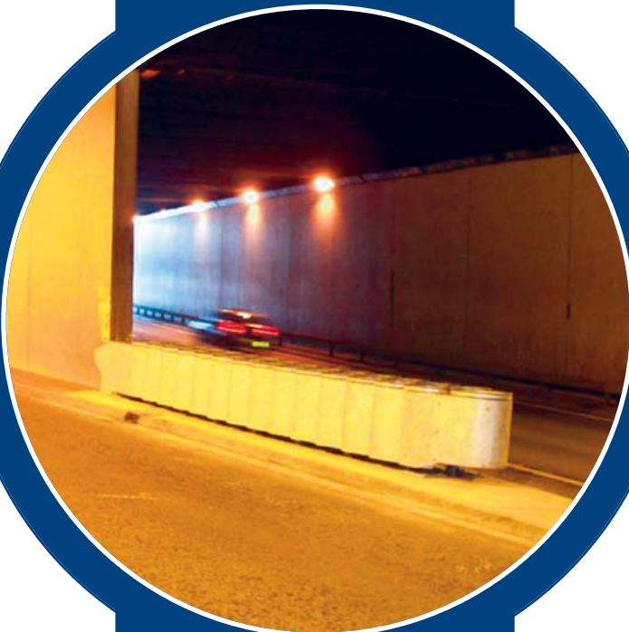
UECL-STOP® crash cushion model P100/2:14 at Charing Cross Underpass, M8 Glasgow.
