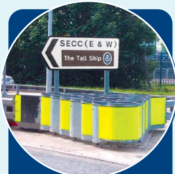
UECU-STOP® crash cushion model V100/5:6 at Ferry Road roundabout A814, Glasgow
