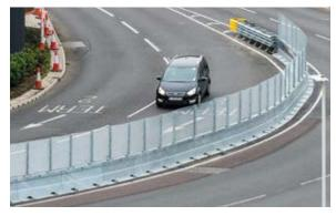
**Zoneguard System 4** is fitted with protective steel mesh fencing (pictured above).
