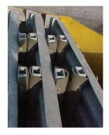
During head-on impacts at speeds up to 110 km/h, the QuadGuard CEN System telescopes rearward, crushing the cartridges and effectively dissipating the energy of both light cars (900kg) and large sedans (1500kg). During angle impacts at angles up to 15 degrees, the vehicles are safely redirected back into the original travel path.
